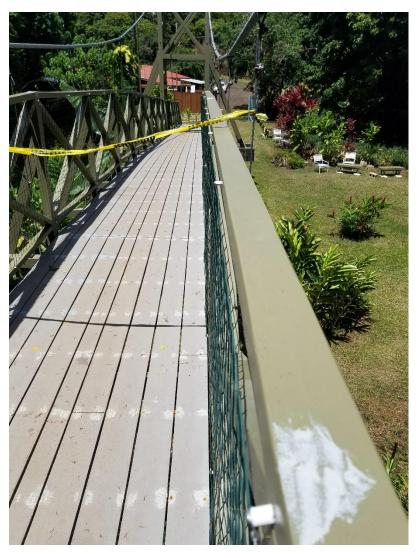
flowers from the walking deck. Periodically, we cut back the overgrowth surrounding the bridge. Still, after 4 years, the structure is in need of preventive repairs. Nails are rusting, some railings are loose and the wire fence guards are coming apart. Our Board of Directors voted to fix the bridge as needed, rather than wait until work becomes major and more expensive. St. John
